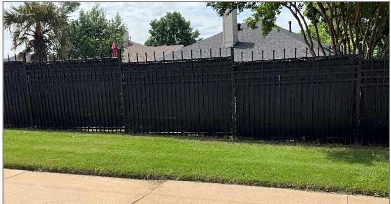
FIGURE 1: EXISTING WROUGHT-IRON WITH TENNIS MESH ATTACHED
